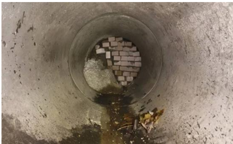
Figure 3-3 Bradley Brook outfall capped
